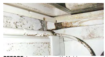
BEFORE: Ice machine with Mold
